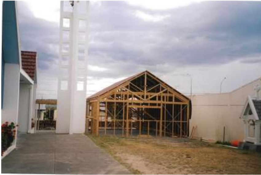
The new Op Shop under construction
