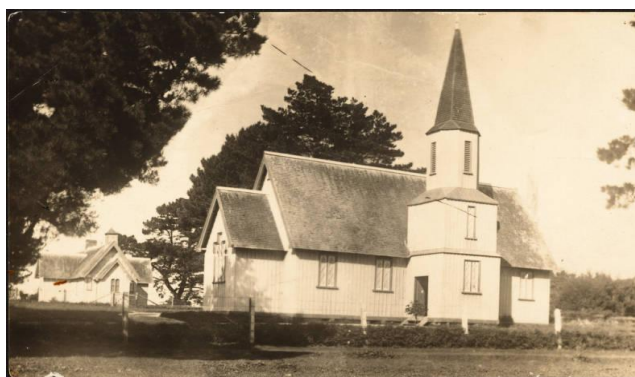
Purchas's second Holy Trinity church on its new Otahuhu site. The original church is just visible in the background, before it was destroyed in the fire of 1912. (This building is now the Selwyn church at Mangere East (AKL Richardson 653-71))
