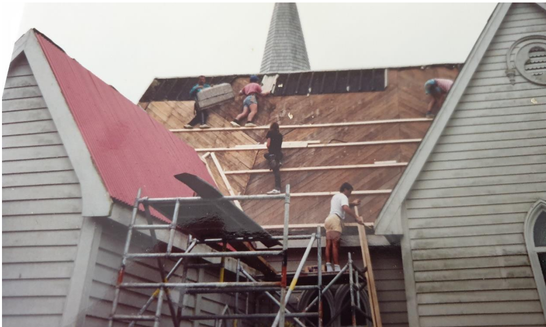
The new roof being installed, the old corrugated iron is on the left.
